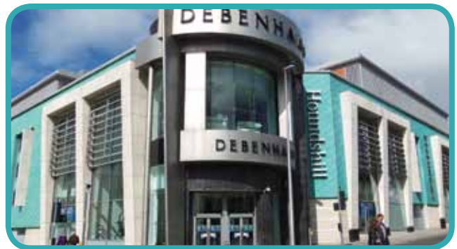
Debenhams Blackpool provided the space for the CP facility, while the council financed the installation and maintenance © John Burke
