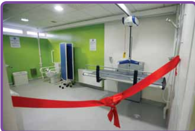
Access to CP toilets provided post-security at East Midlands Airport
