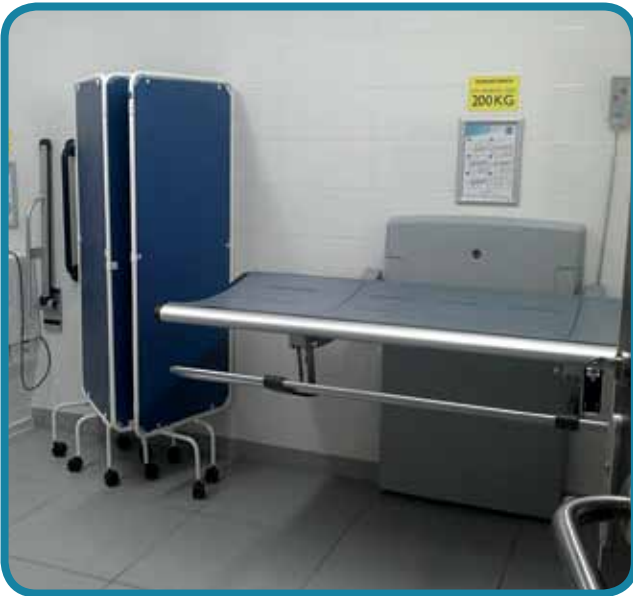
A wall-mounted changing bench at Cherwell Valley Moto Services. It is height adjustable, with maximum-load capacity and instructions clearly on display
