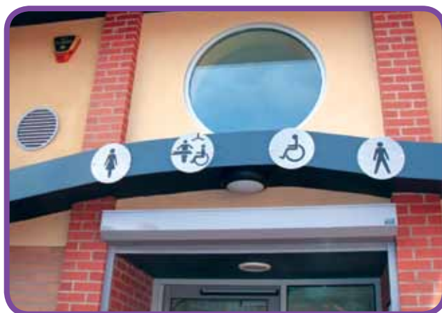
Visually contrasting symbols and non-reflective signage at Newark town centre's public toilet facilities. Opening hours are extended to cater for events
